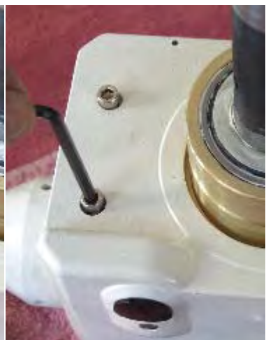
Tigytan the cap headed screws down but not too tight.
