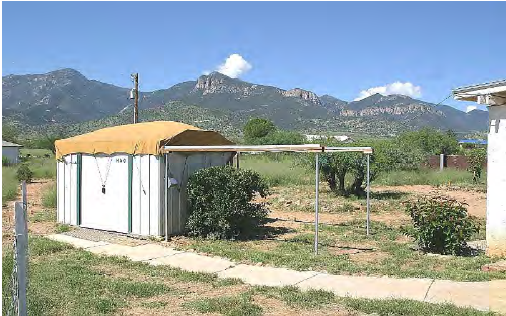
Figure 2.01 “Hereford Arizona Observatory” with a canvas-covered sliding roof. The Minor Planet Center has assigned it a site code of G95.
